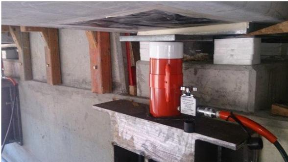
A 20mm support plate was placed on top of the jack to evenly distribute the load and these were grouted with fast curing Chemrite CR-FC grout.
