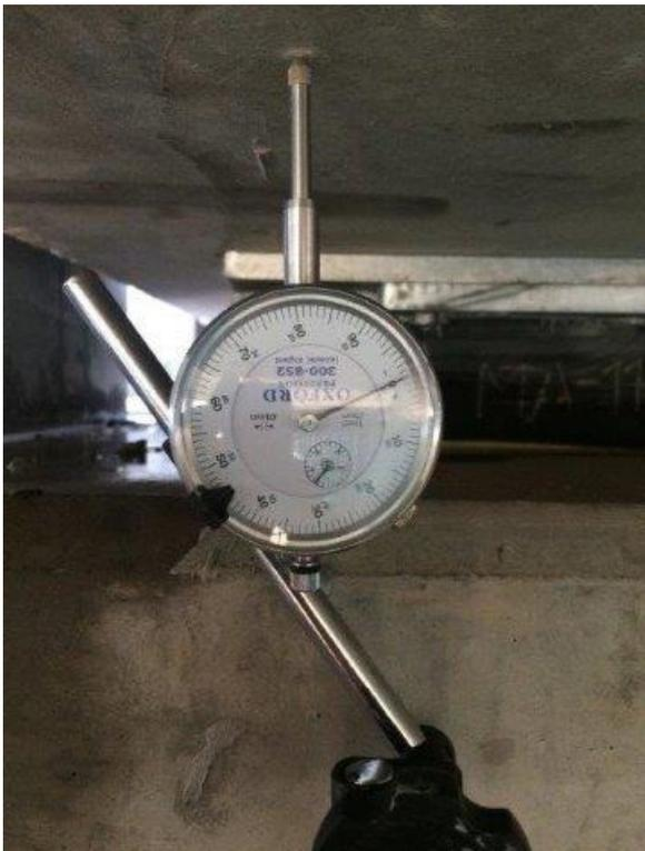
Each girder was then lifted to a point where each bearing could be removed. This was done using basic hand tools and much care was taken not to damage the elastomeric bearings.
