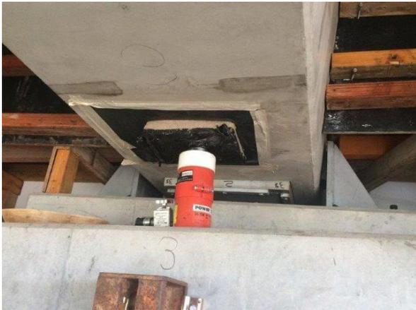
A 20mm support plate was placed on top of the jack to evenly distribute the load and these were grouted with fast curing Chemrite CR-FC grout.
