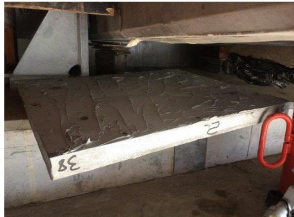
Once the taper plates were removed, they were cleaned and replaced with epoxy grout and new HD bolts.
