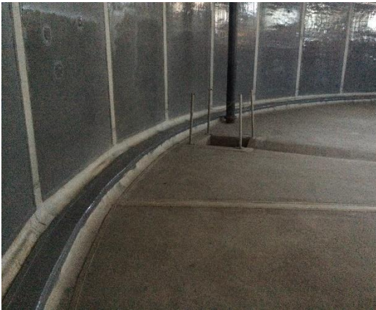
Reservoir walls and ringbeam coated with Tufflon P-90 (Polyurea coating).
