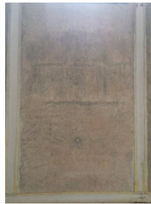
Remove existing coatings (After)
