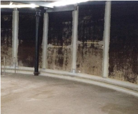
Remove existing coatings (Before)
