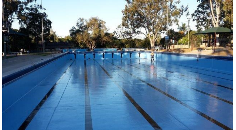
Ferny Hills Pool –Scum Channel and coating completed
