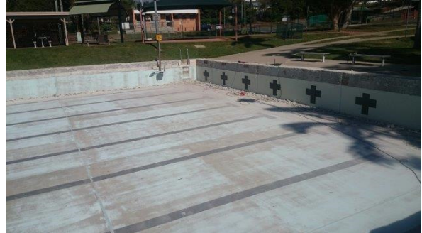
Ferny Hills Pool –Scum Channel and coating completed
